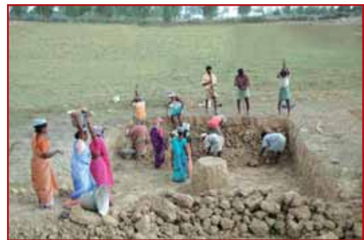
Desilting at Kollafarm tank, Chittoor Dist., Andhra Pradesh
