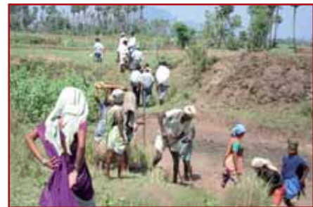
Vijaynagaram work site, Andhra Pradesh
