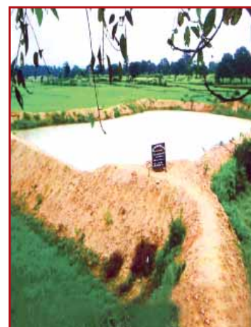
Construction of pond in Turubul, Dist. Gumla, Jharkhand
