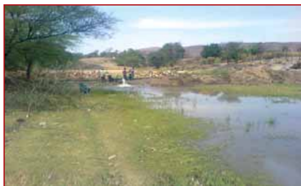
Strengthening of canal, Dungarpur, Rajasthan
